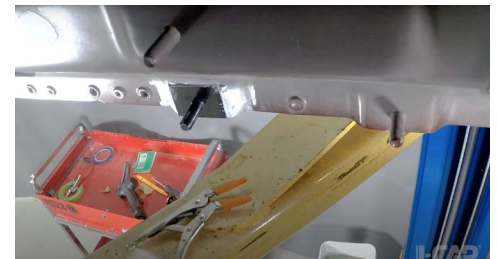
The near-finished repair with the new attachment in place.
